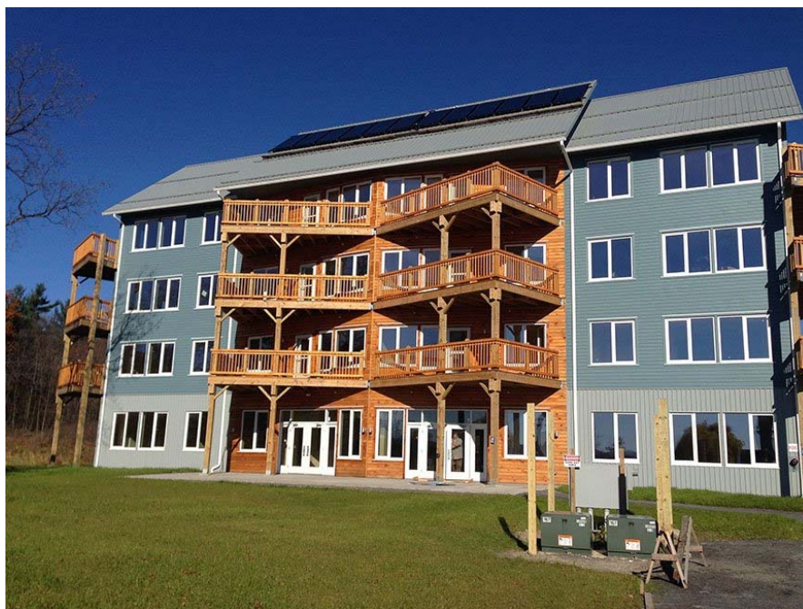
Figure 7. The Sustainable Living Center at EcoVillage South wall
